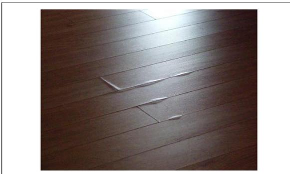
Fig. 1 : Example application of MDF: flooring, having suffered water damage.
